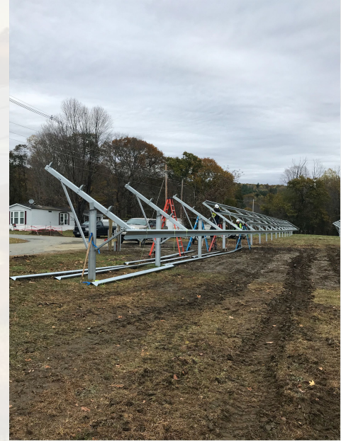
Building the Array (Oct. 29, 2018)
