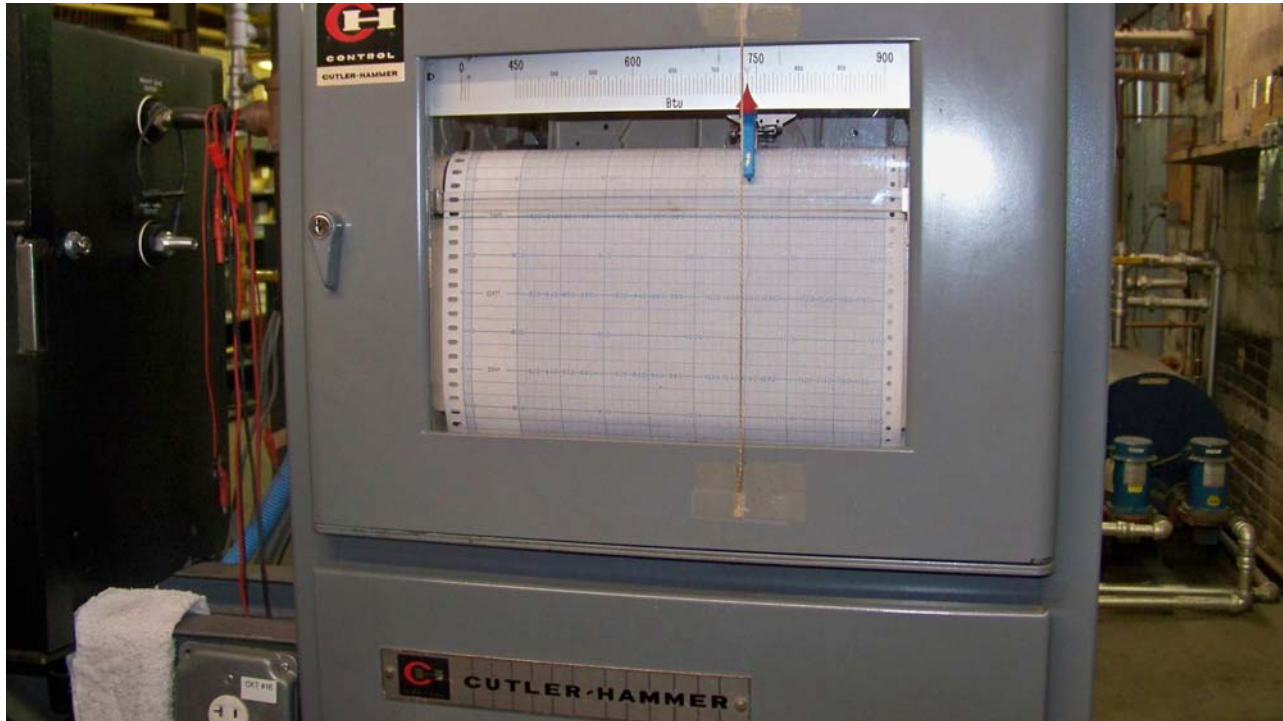
Liberty Keene – The plant propane/air output Btu heating value is monitored and recorded using a Cutler-Hammer calorimeter.
