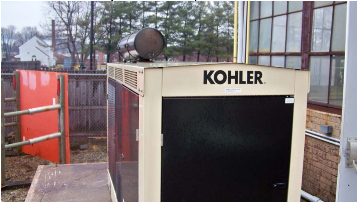
Liberty Keene – The air blowers are equipped with a 125 KW emergency generator.
