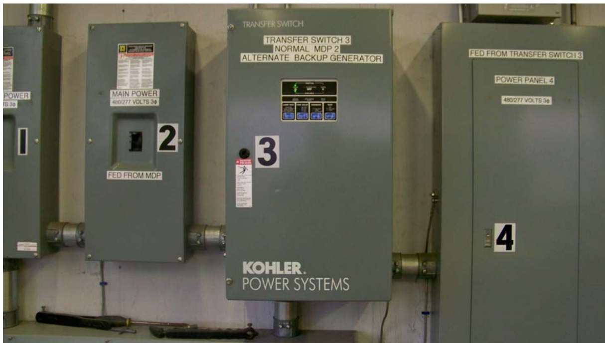
Liberty Keene – The system was not configured to transition to emergency backup power without experiencing a brief power interruption to the variable speed drives which requires manual restart of the blowers.
