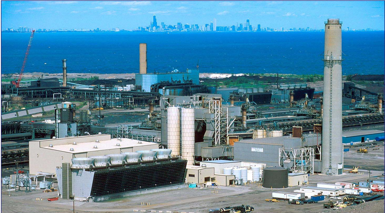
Figure 1. Cokenergy - Energy Recycling Plant at Mittal Steel, East Chicago, Indiana
